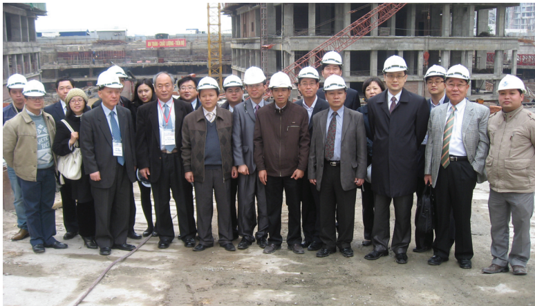
Construction Site Visit (Vietnam Mission)
